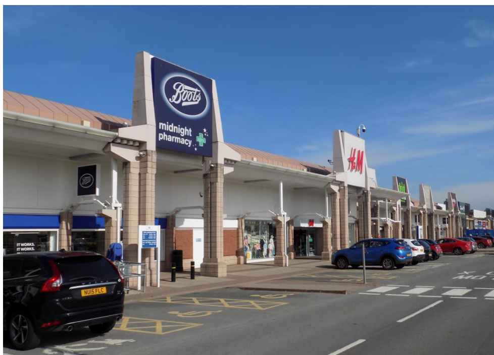
Figure 2.12 Teesside Shopping Park
