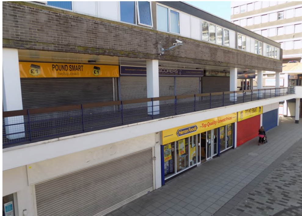
Figure 2.6 Vacant Units, Queensway
