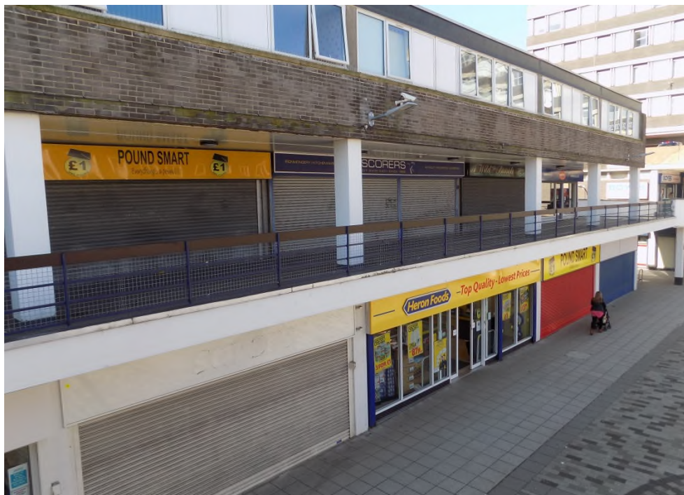
Figure 5.4 Units on South Side of Queensway
