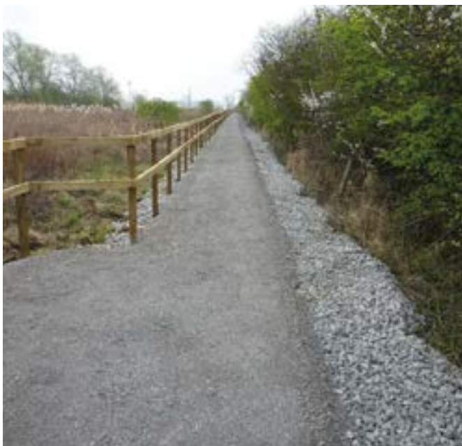
New Causeway (view towards Brine Pumping Station)
