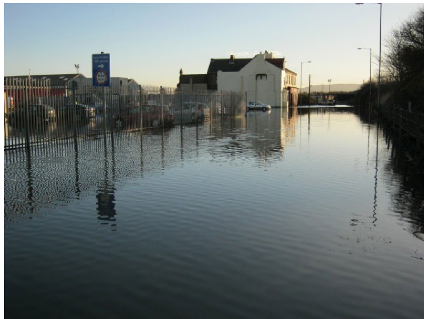
Port Clarence - Calor Gas Site
