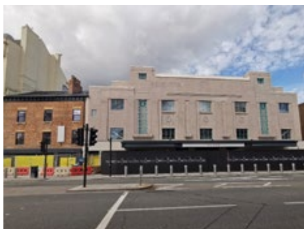
Photograph: Globe Theatre, under construction 2021
